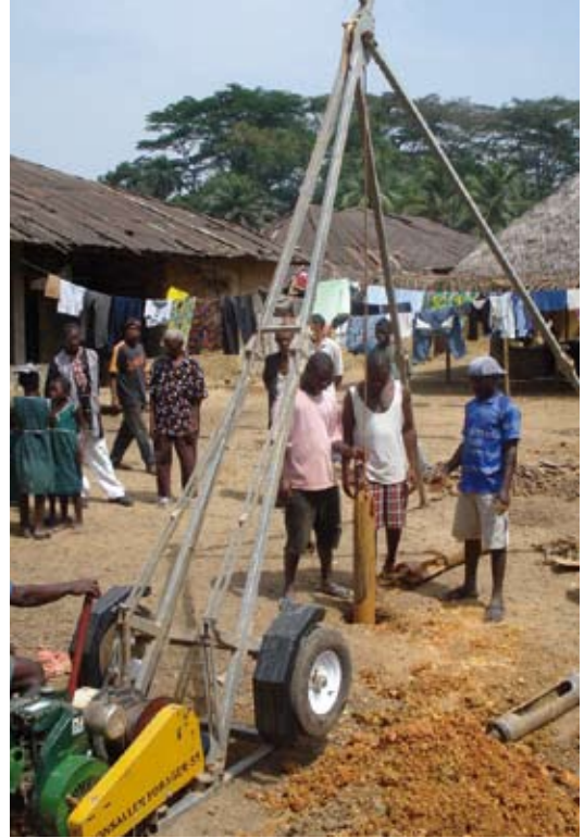
Drilling for Water, Pujehun
